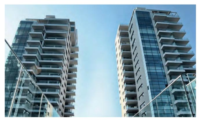
A pedestrian bridge over the beach road connects the 2 towers with the beach. The building envelope of both towers is constructed using reinforced concrete and it is decorated throughout with stone, aluminium and glass.
