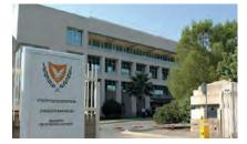
The building is a 5-storey reinforced concrete structure. Its facilities include executive offices separated by demountable partitions, conference rooms, an auditorium, libraries, computer and storage rooms. All the external cladding of the building consists of a curtain wall and granite. The infrastructure works comprised of roads, parking facilities, street lighting and extensive well-made outdoor landscaping.
