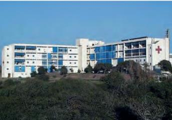
The exterior works of the contract included repairs to the concrete facades using high pressure jetting techniques and specialised concrete materials. The interior works included extensive refurbishment works throughout the hospital. Other works of the contract included the installation of new lifts, the replacement of boilers, calorifiers, pumps and distribution pipework and the installation of piped medical gas distribution systems.
